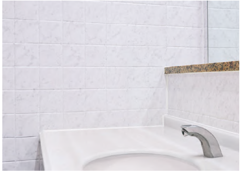
Restroom refurbishment / ST-024TIL
